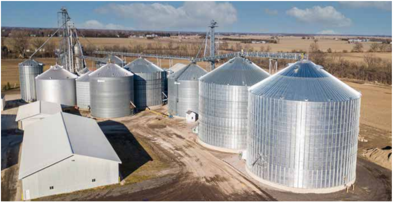
John Marion, Inc.'s branch elevator outside of Britton, MI, with new 400,000-bushel Behlen tank at far right. Drone photo by Raines Aerial Photography, Wapakoneta, OH.
